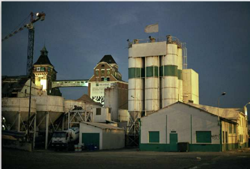
Cimenterie // Cement works
